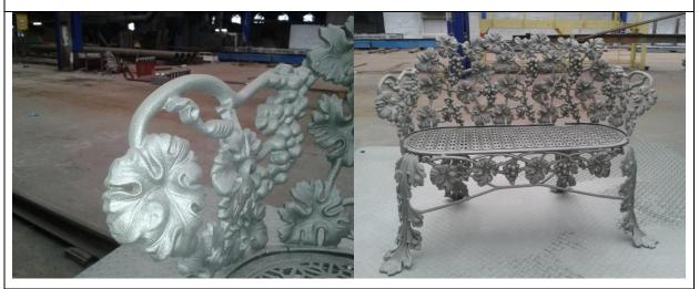
Once in a blasted state and free from contamination we appllied 125 microns of a Zinc Phosphate primer. This coat is designed to give anti-corrosive protection to the iron underneath. Due to the complex nature of the bench the painter was required to brush in a stripe coat before the appliaction of the full coat by airless spray.
